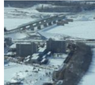
New bridge construction will help relieve traffic congestion in Fort McMurray
